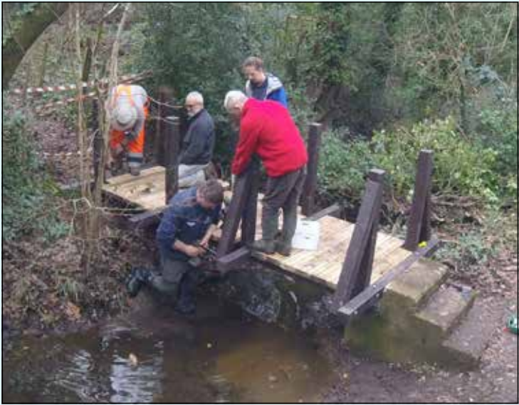
Work in progress. Photos: Martin Dunn
